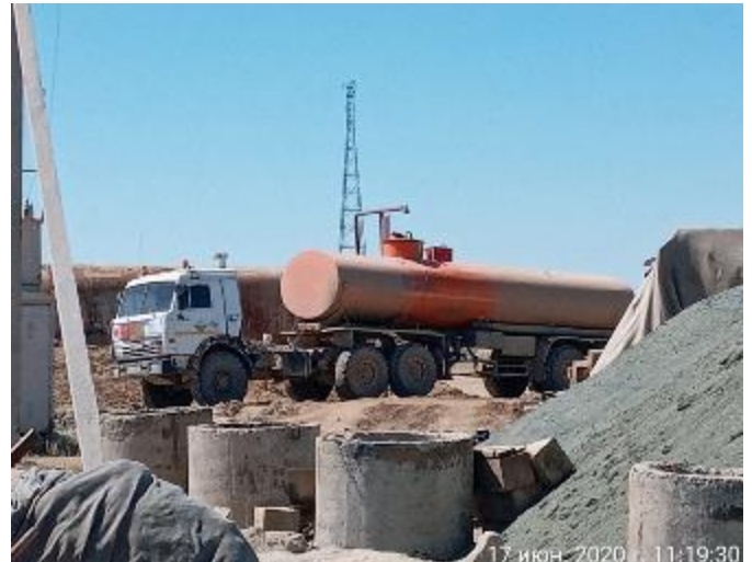
Audit on 17.06.2020, reinforced concrete rings for arranging a septic tank for collecting liquid waste
