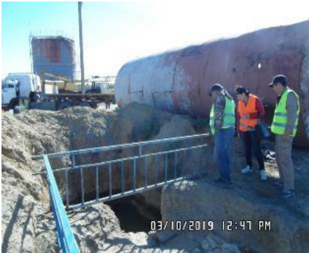
Audit on 03.10.2019, unorganized runoff of liquid waste.
