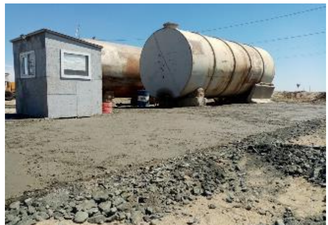
Concreting of the site under the storage tank for fuels and lubricants, Production base in Karaulkeldy village, Audit in May 2020.
