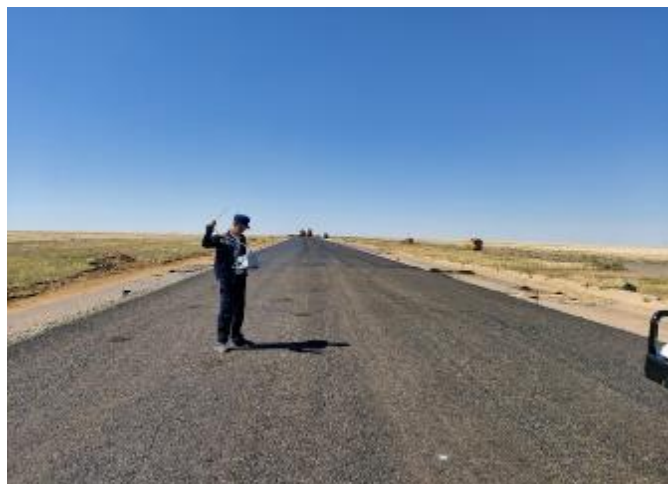
Measurements of noise and vibration level on lot 3
