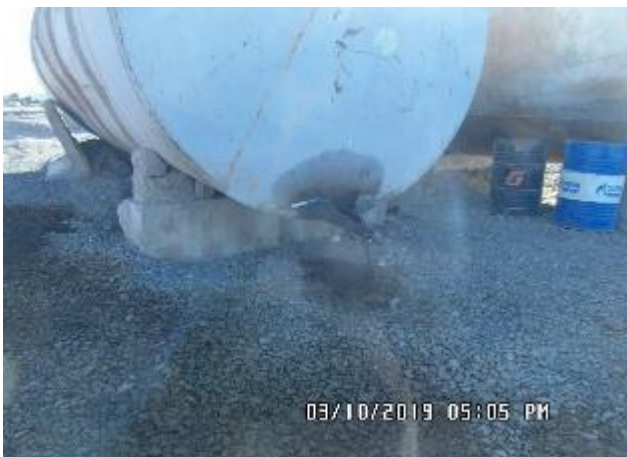
Spills at the storage site for fuels and lubricants, Production base of Karaulkeldy settlement, Audit in October 2019
