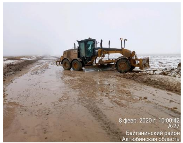
Leveling by grader on Lot 3
